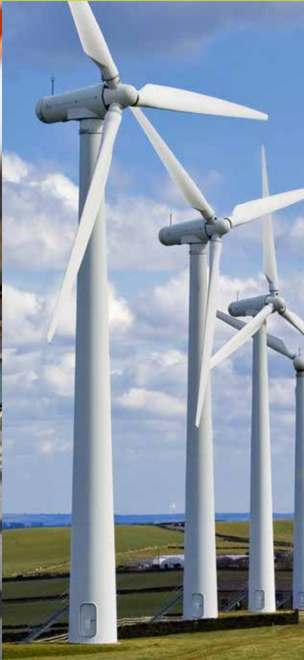
MACHINE AND SYSTEMS ENGINEERING
